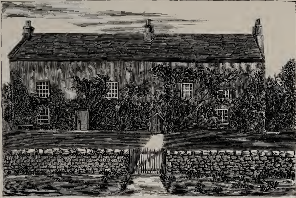
OLD WEST LAYTON HALL.
