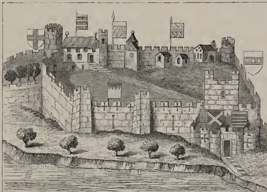
THE CASTLE OF RICHMOND AFTER IT HAD BEEN REPAIRED AND ENLARGED BY EARL ALAN 1ST, AND BEFORE THE GREAT KEEP WAS BUILT.
